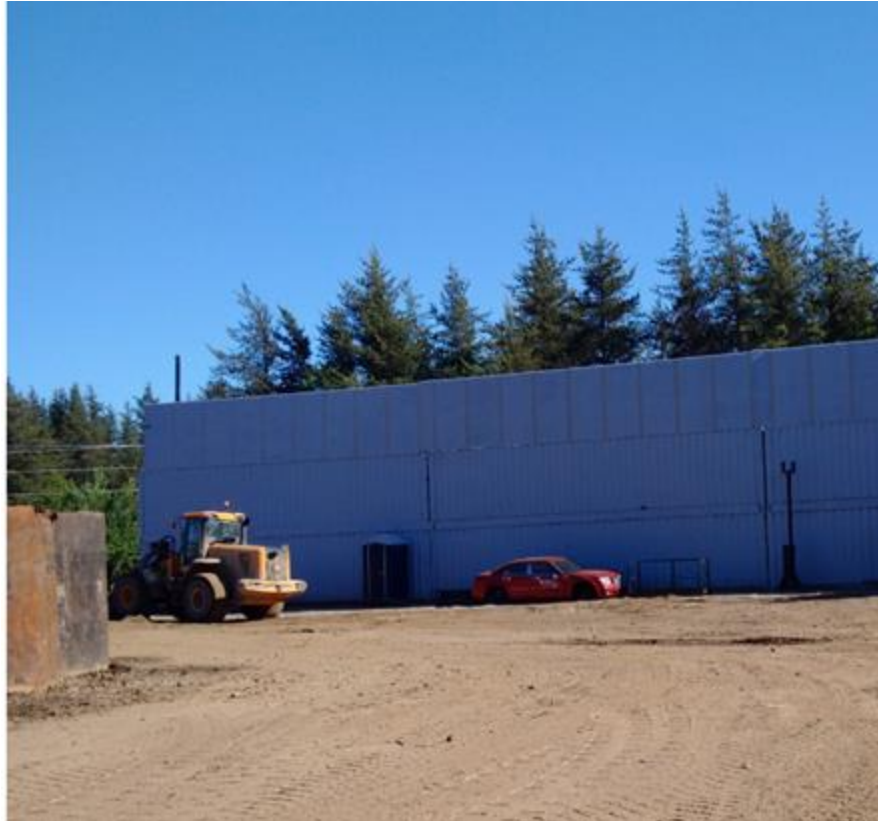
Figure 2 Shipping Container-Based Barrier – Front
