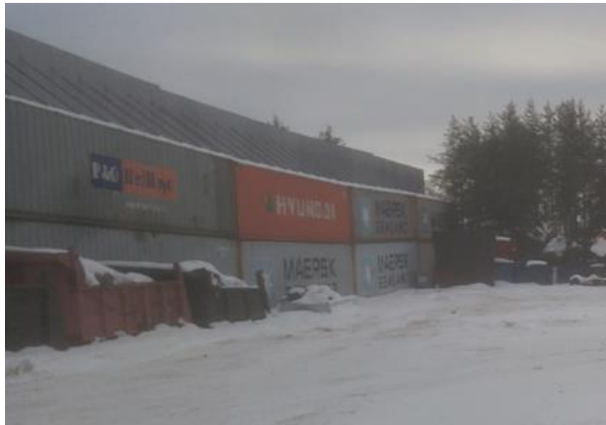
Figure 3 Shipping Container-Based Barrier – Back
