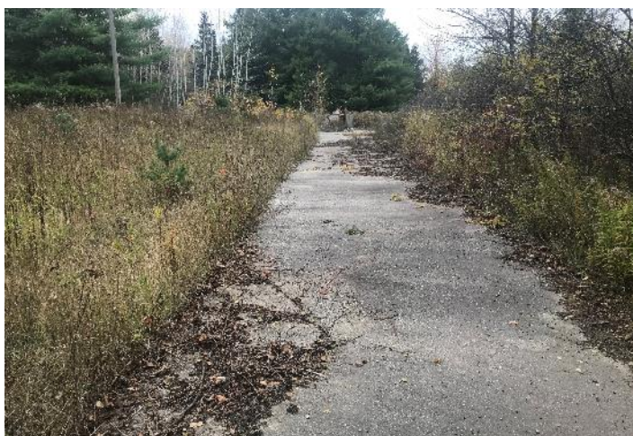
Image 14: CBM Lanci Stage 2, driveway to abandoned/demolished home, facing west.
