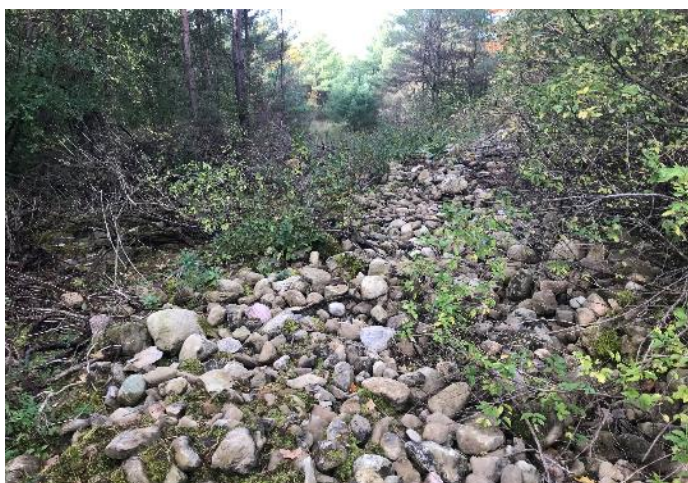
Image 26: CBM Lanci Stage 2, area of rock rubble disturbance, facing west.
