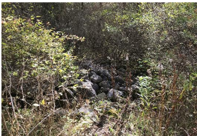
Image 33: CBM Lanci Stage 2, piled stone before area of steep slope, facing east.
